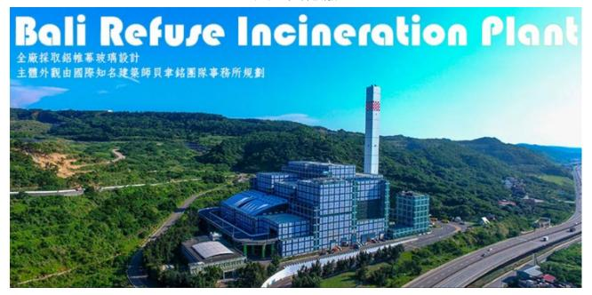
Bali Refuse Incineration Plant is located in Bali District, New Taipei City. It processes about 400,000 metric tons of both household waste and industrial waste per year and converts them into electrical energy. The annual power generation capacity is about 250,000 MWh, which performs highest energy conversion efficiency among 24 incineration plants in Taiwan.
